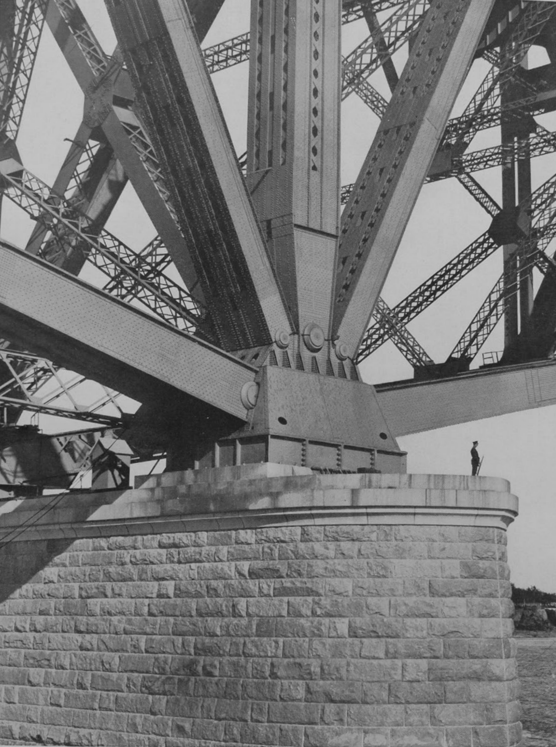
View of Main Truss Members pin connected to the shoe
