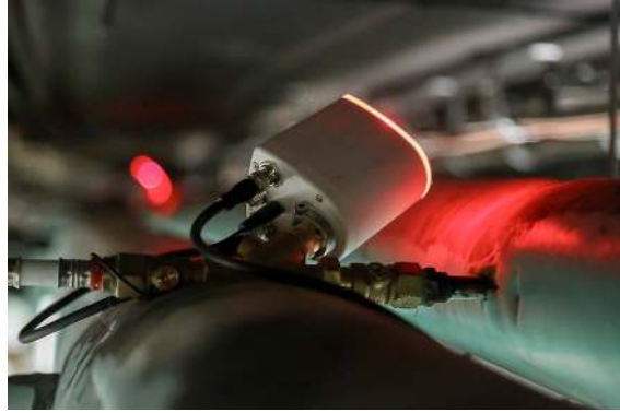
When all 72 valves were installed, connected to two system masters and a control unit, and after a first automatic adjustment, the system functioned flawlessly.
