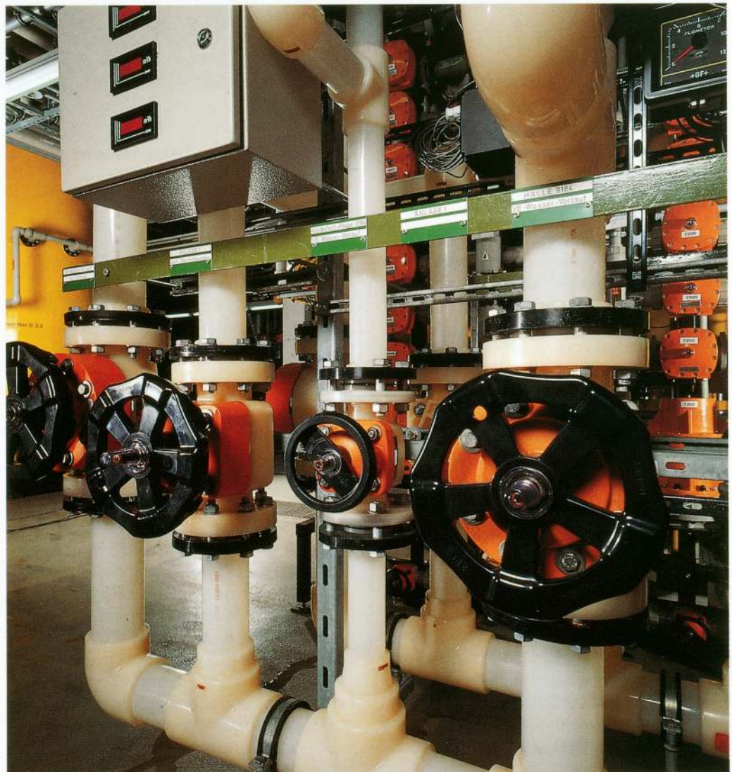
A SYGEF®-HP (High Purity) piping system in the semiconductor industry. High-purity water distribution and metering for the manufacture of large-scale integrated semiconductor components
